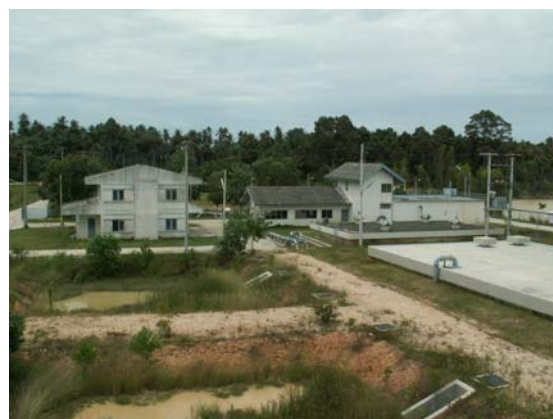
Figure 7. Water treatment plant at Na Muang
