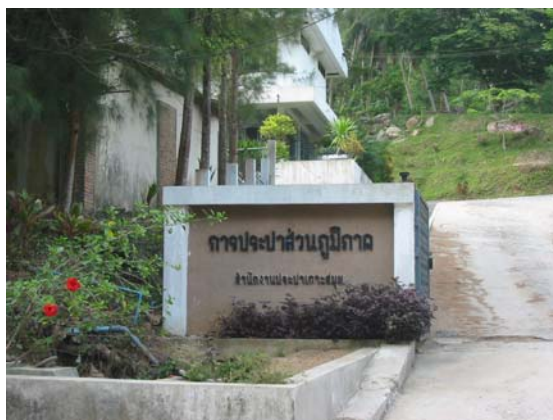
Figure 6. Water treatment plant office at Hin Lad
